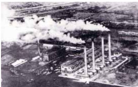
Fukagawa Incineration Plant (1933), Capacity: 940t/day
